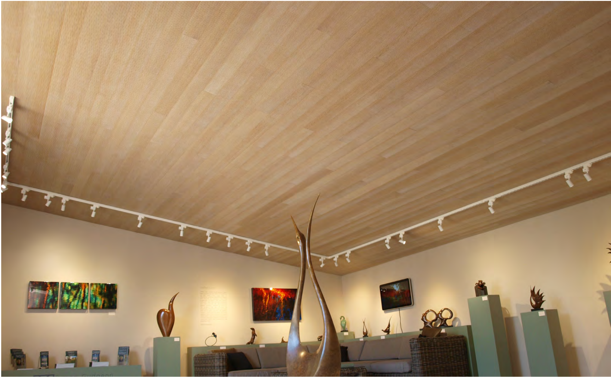
TOPLINE 6/2 ACOUSTIC CEILING PANELS IN WHITE-WASH HAND-SPRAYED FINISH, KEEPING THE CONSISTENCY WITH THE GALLERY'S NATURAL CONTEXT
