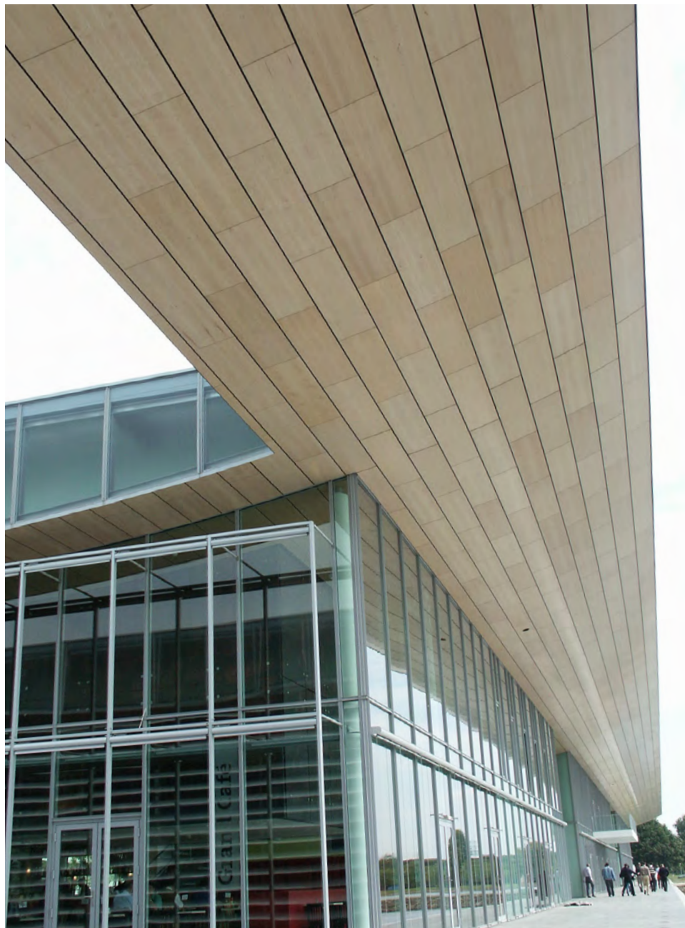
LAWAPAN STANDARD CEILING PANELS: INSTALLED TO BOTH INTERIOR AND EXTERIOR, IN A CONTINUOUS CEILING CONFIGURATION
